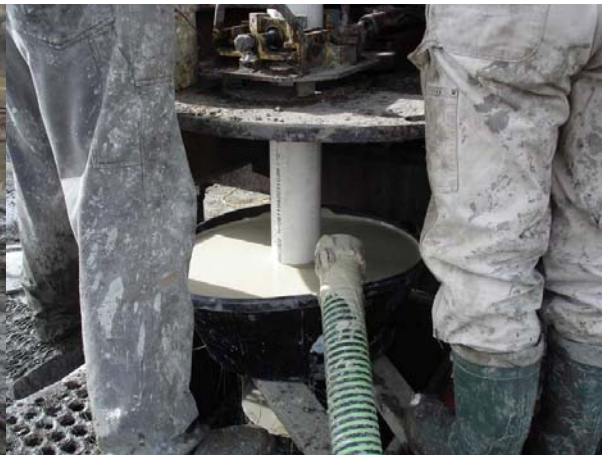
Installing and Grouting Liner
