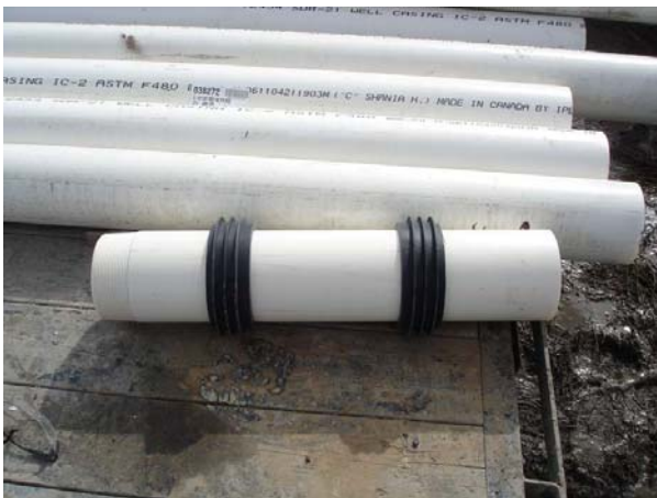
K-Packer on Casing Liner
