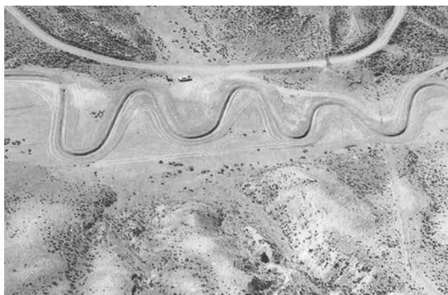
CBM Ditching on Maycock Ranch
