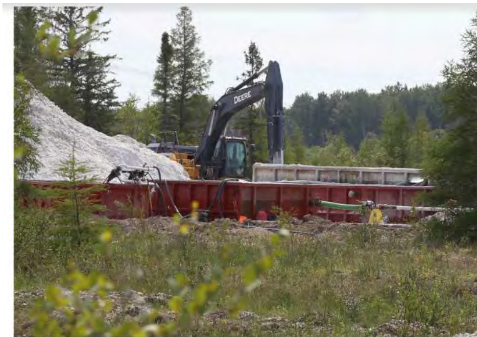
Figure 5. CWS sand extraction activities in a quarry site near Vivian MB Aug. 18, 2021
